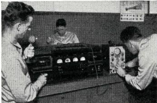
Checking performance of a radio-telephone transmitter with an oscilloscope. National trained Radio Technicians, in Broadcasting Stations, in Industrial Plants and in business for themselves are well paid specialists. Their services are in urgent demand.
