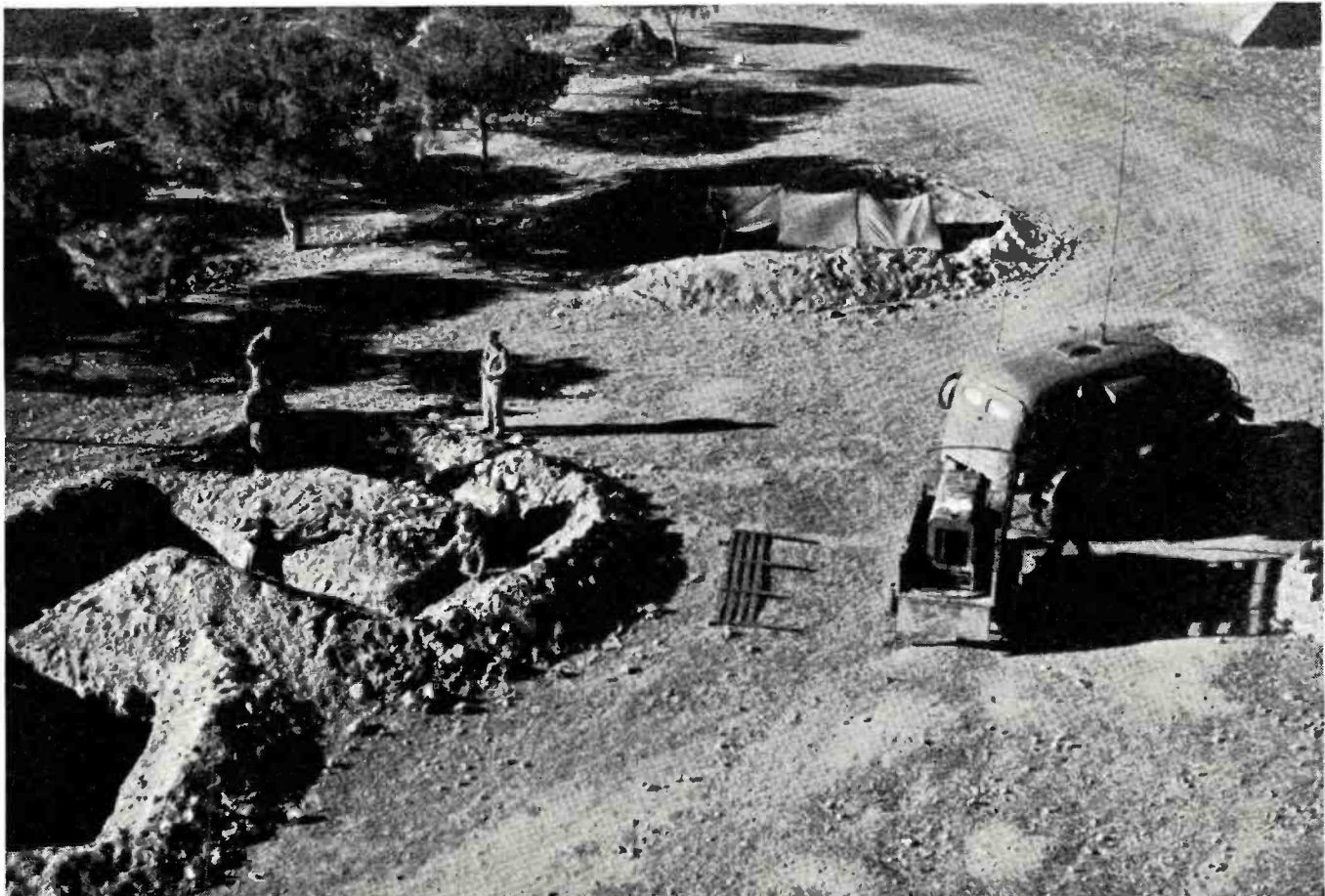
Members of U. S. Aviation Engineers building shelters near air field in Youks Les Bains, North Africa. SCR-299 on right.
