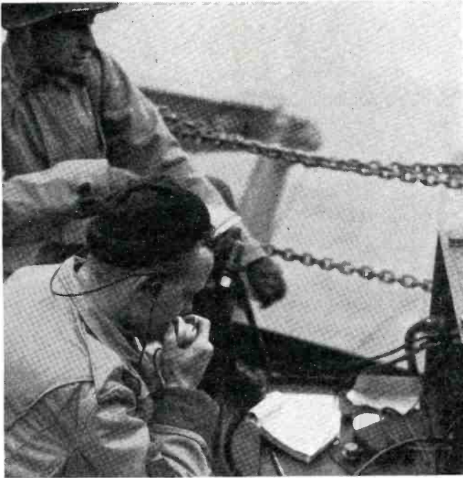
Maintaining contact with first wave as it lands on Attu.
