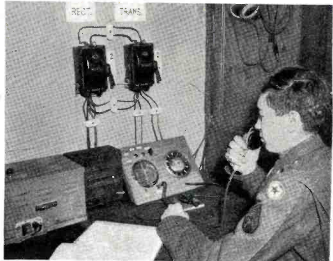
Control station showing receiver and transmitter control panel.
