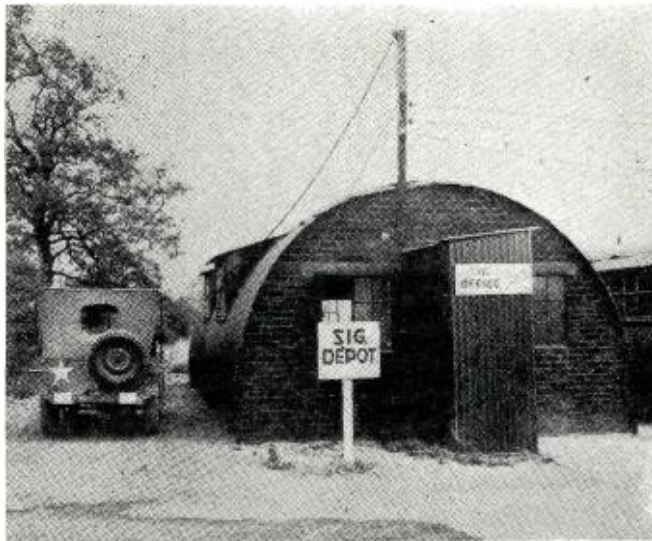
Office of a typical Signal Depot—a quickly erected Nissen hut but used widely in the European Theater of Operations.
