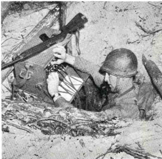
"Dig your switchboard in early" is the cardinal principle in all amphibious training. Communications are vital in any offensive.
