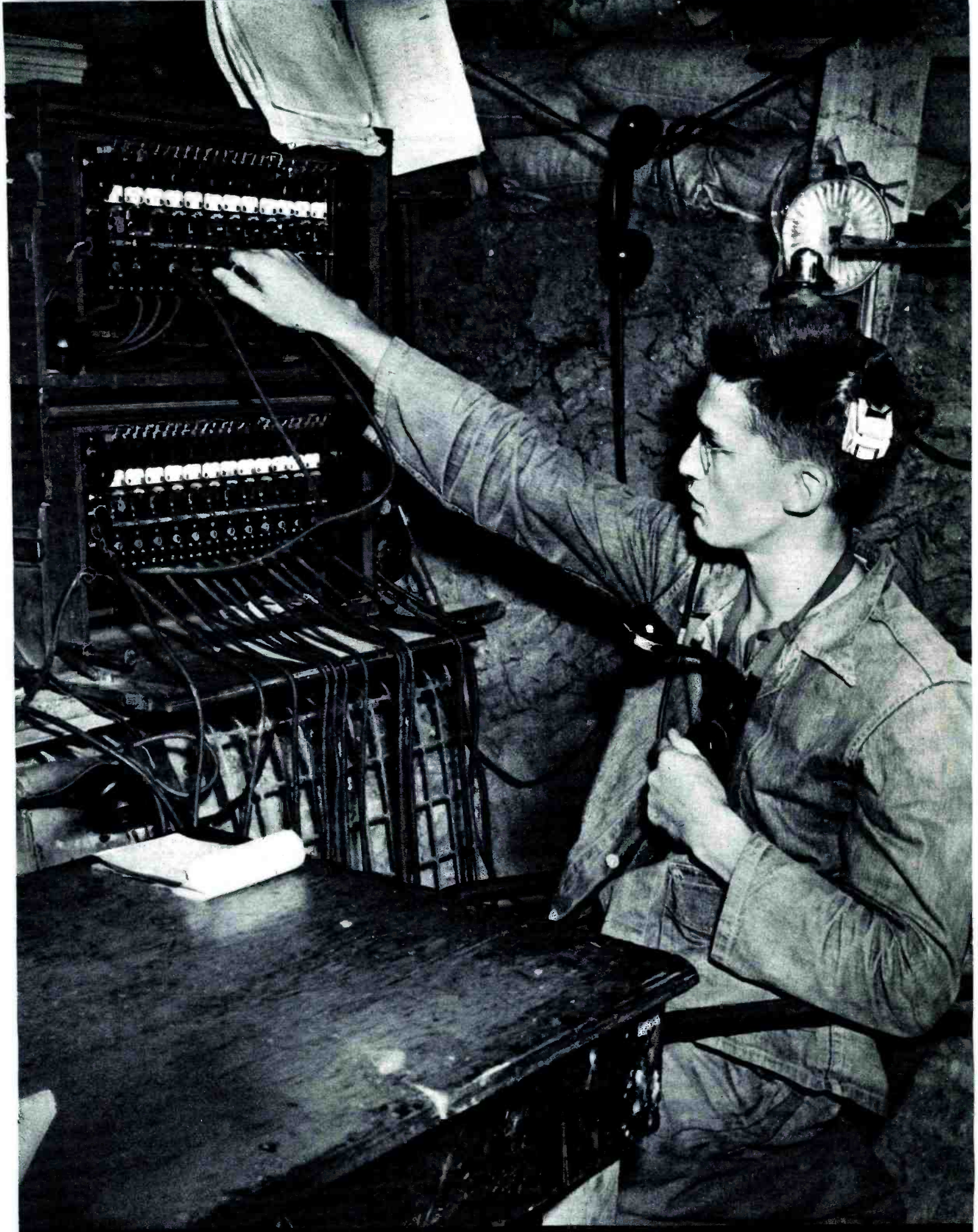
Pfc. Edward C. Griser operating the BD 72, 12 drop switchboard in a communications dugout somewhere in New Guinea. www.americanradiohistory.com
