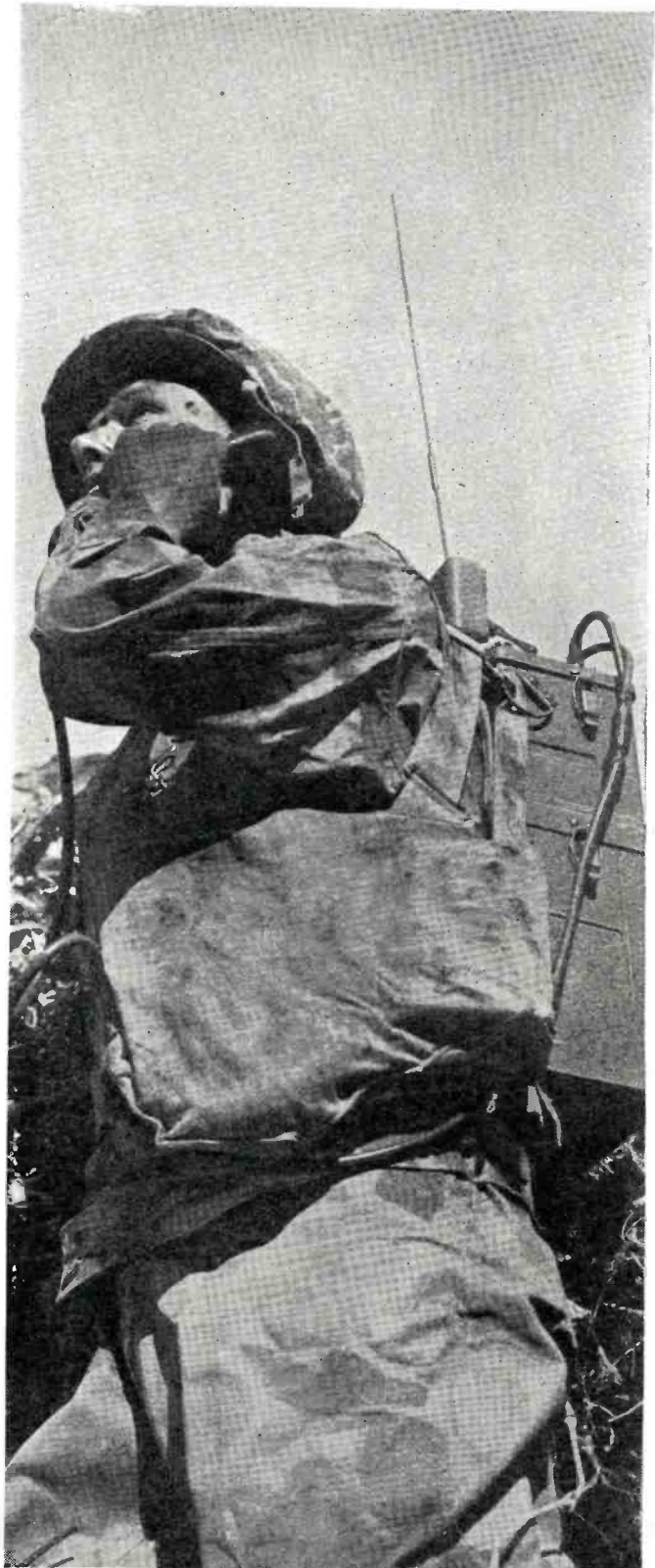
Moving through dense underbrush with the Army's powerful one-man radio set—the FM walkie-talkie. Weighs 35 pounds complete.
